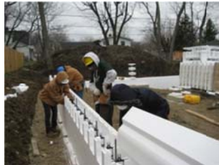
INSTALLING INSULATED CONCRETE FORMS
